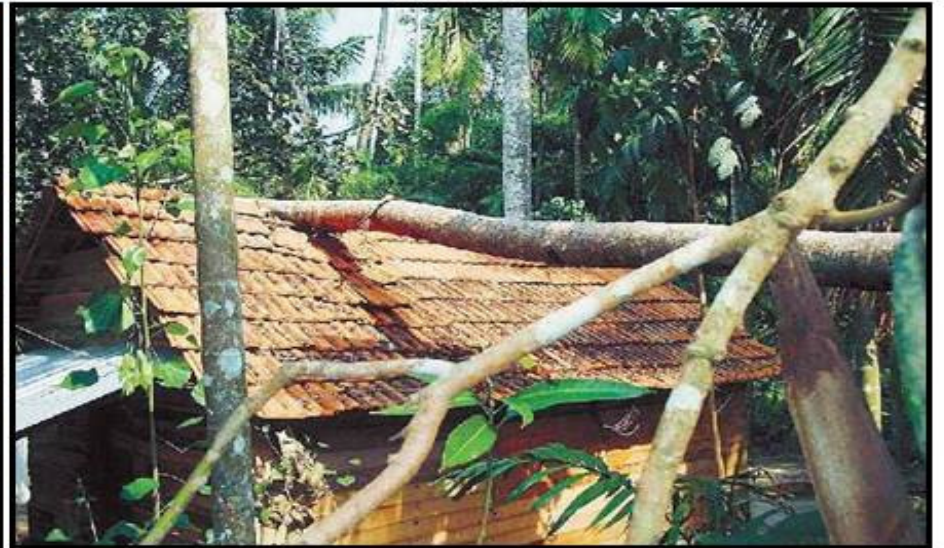
Damaged house due to tree collapse at Kulasekaram, Trivandrum 16.04.2014
