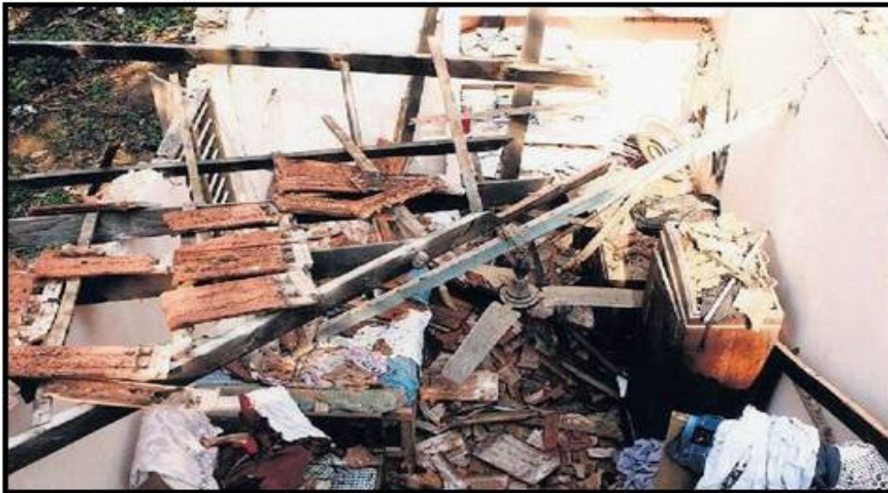
Completely destroyed at Kalarithara, Kottayam 15.04.2014
