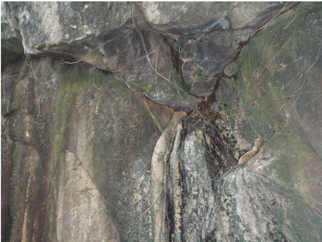
The highly fractured joints probably with no anchor
