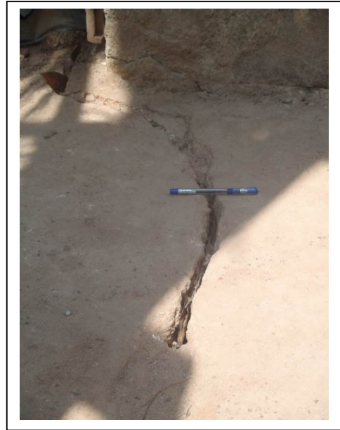
Figure 12: Curvilinear extension of ground fractures
