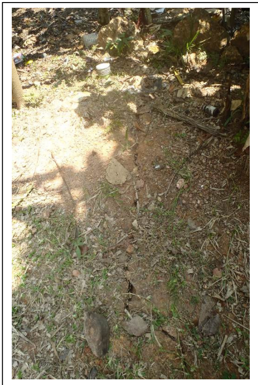
Figure 17: Continuous extension of ground fissure seen in the Eastern side of the valley
