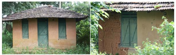
Figure 9-19: A typical unit in the projectFigure 9-18: Exposed walls with cracksThese houses were built based on sustainable housing concept. Rammed earth constructiontechnology was used for the basement and foundation and cob construction for the walls.Hard wood was used for the construction of windows and doors. The houses were plastered
