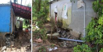
Figure 6-3: Scouring of foundation soil
