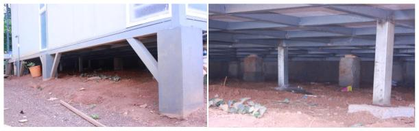
Figure 9-10: The load bearing stilts in foundation
