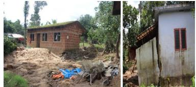
Figure 6-2: Partially Damaged- dislocation of wall masonry
