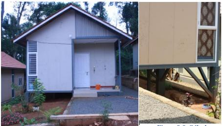
Figure 9-9: A typical V panel unit
