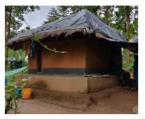
Figure 3-7: The two level foundation of an indigenous house
