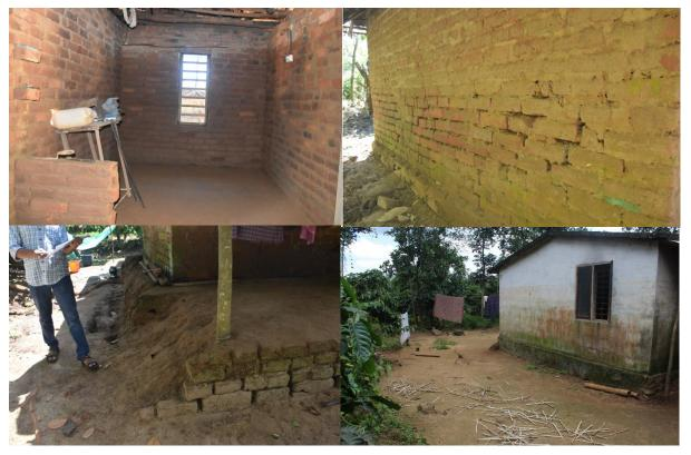
Figure 5-8: Pattern of damages due to flood
