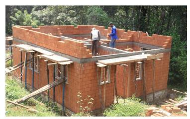
Figure 9-17: An interlocking mud block unit under construction
