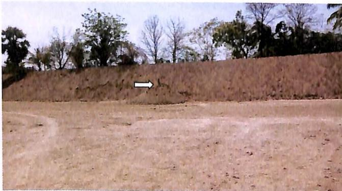
b) Another view of the completed bund without grass cover. Note the small mound in the foreground with a PVC pipe in the centre. This is to record the ground water level in the pond. Total height of the pipe is 7.6 m.
