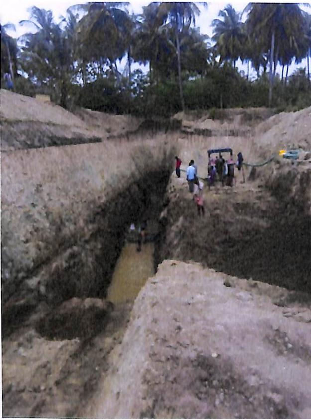
Figure: 17b. Further progress of excavation in the northern part. The depth of excavation has reached about 7 m from the original floor level of the pond. The dark layer in the bottom part of the trench shows weathered rock. Water is being pumped out of the trench using a tractor mounted heavy duty pump.
