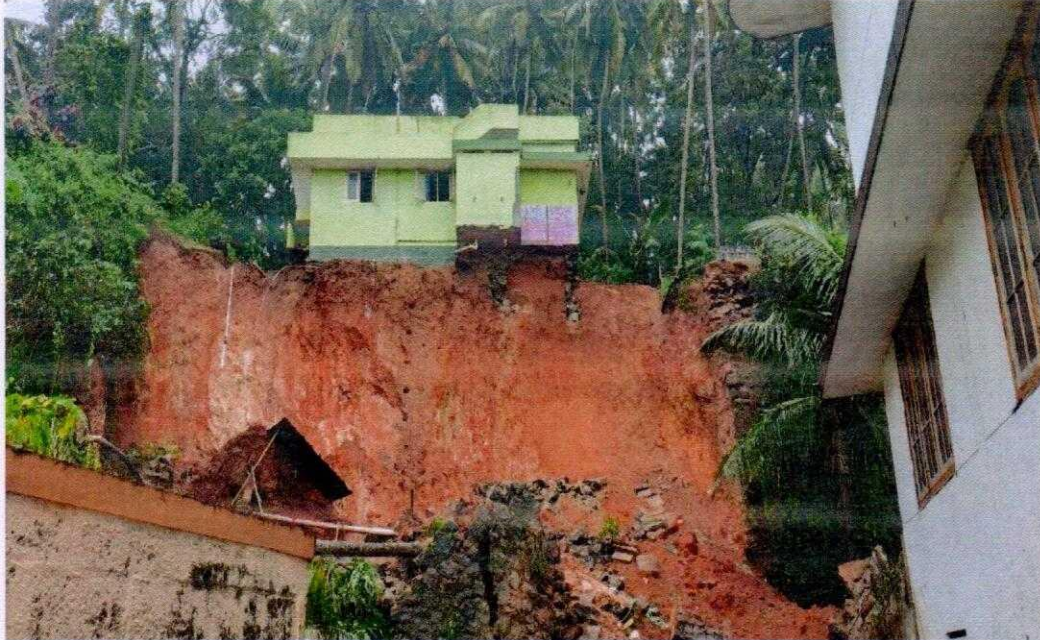
Damaged Retaining Wall and Breast Wall
