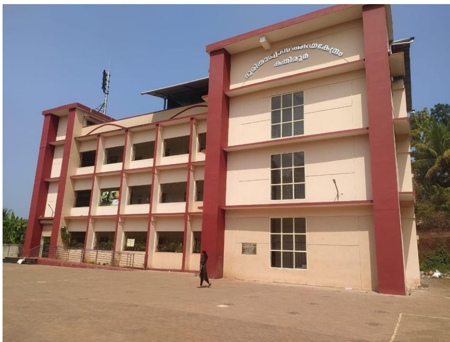
Figure 7: Multi-purpose Cyclone Shelter, Kathiroom, Kannur
