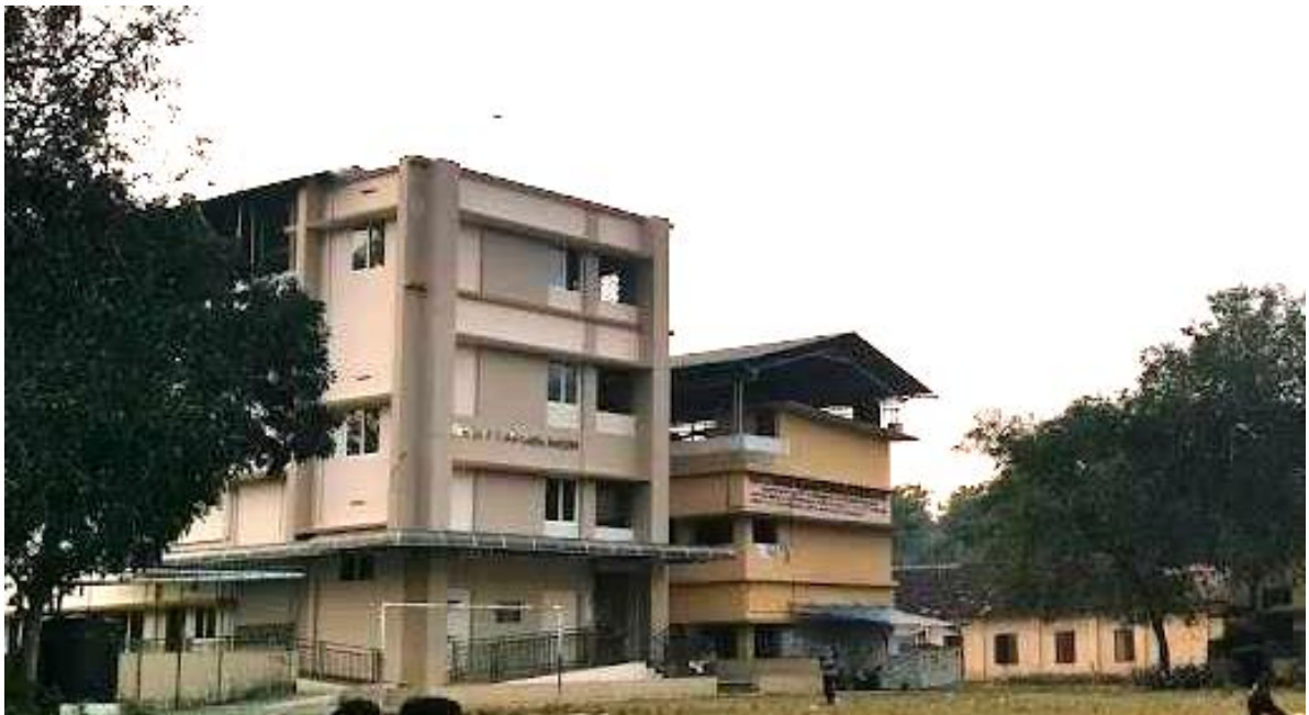
Figure 16: Multipurpose Cyclone Shelter, Cheruthana, Alappuzha
