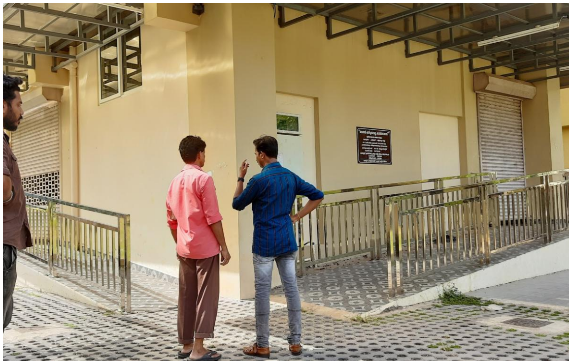
Figure 18: Ramp for wheelchair access
