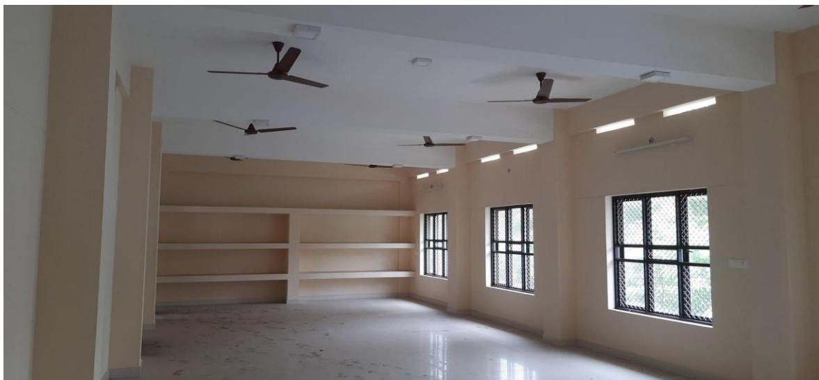
Figure 30: Existing space in common dormitory in MPCs
