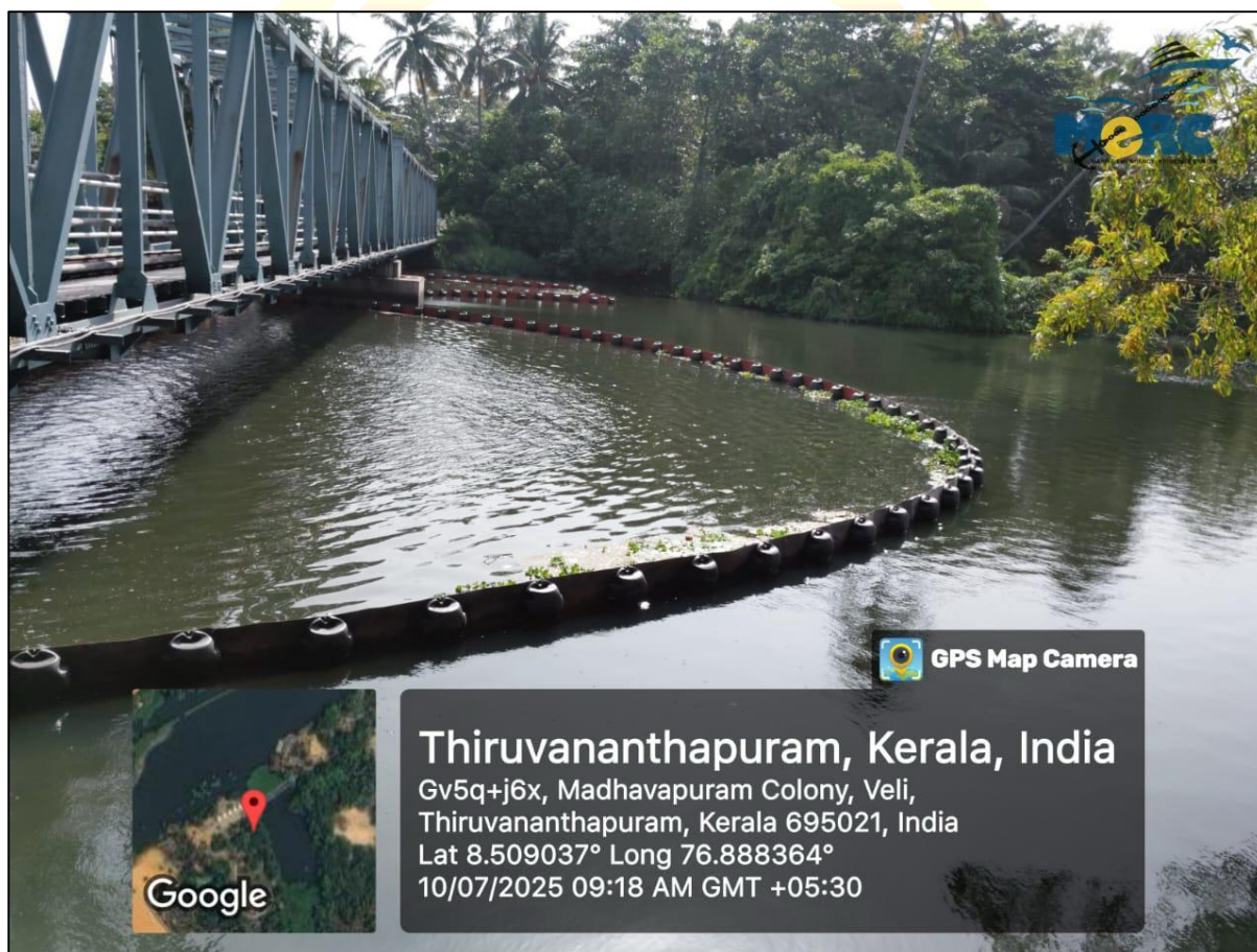
Figure 2: Deployment of booms
