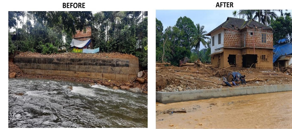
Figure 8-8: Protection wall before and after landslide
