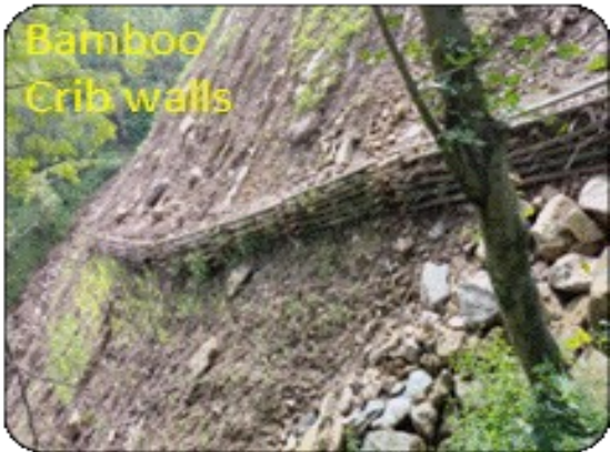
Figure 9-4: Bamboo Crib walls
