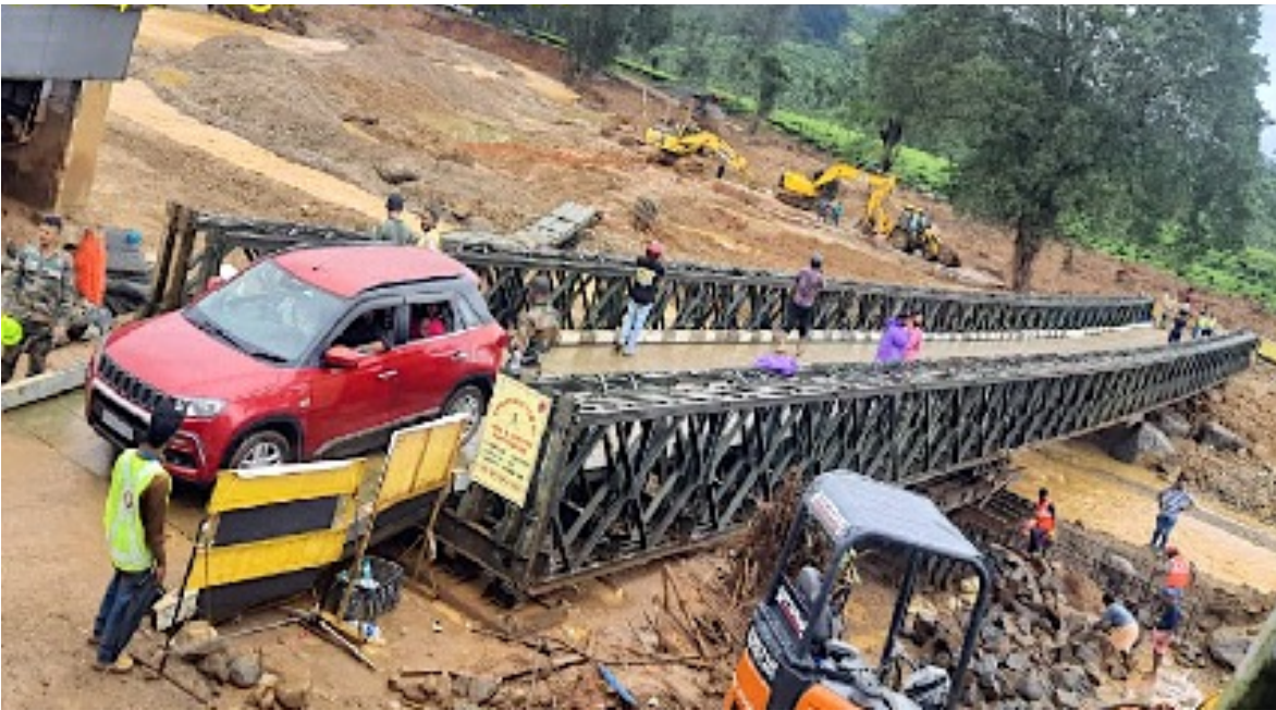
Figure 9-3: Bailey bridge constructed at Chooralmala by Army
