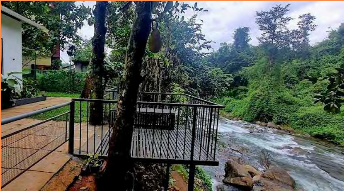
Figure 13-3: Linora Service Villa before landslide
