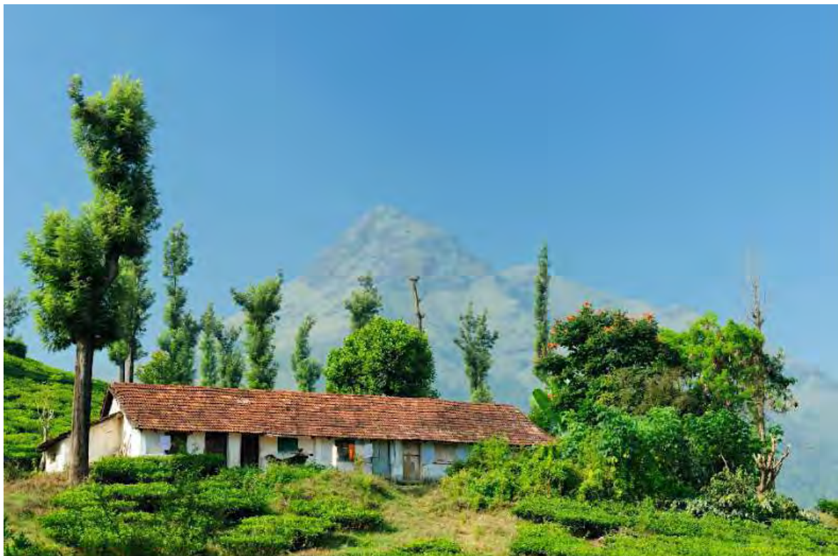
Figure 2-1: Padis – Line Quarters (before landslide)
