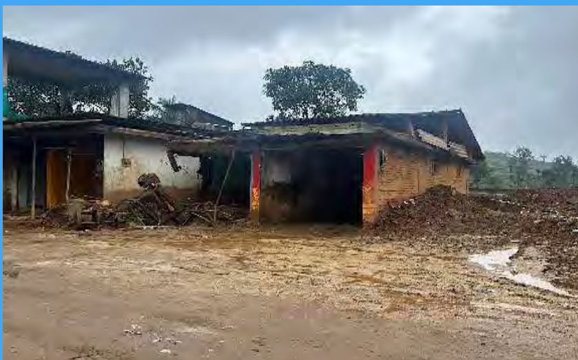
Figure 5-3: Damaged ration shop at Chooralmala
