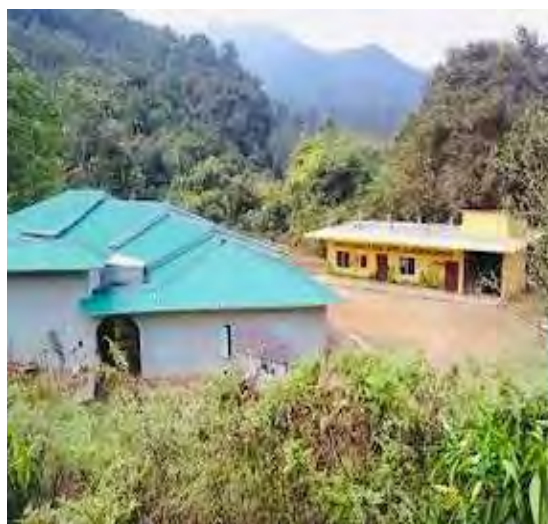
Figure 4-5: GLPS Mundakkai before the Landslide
