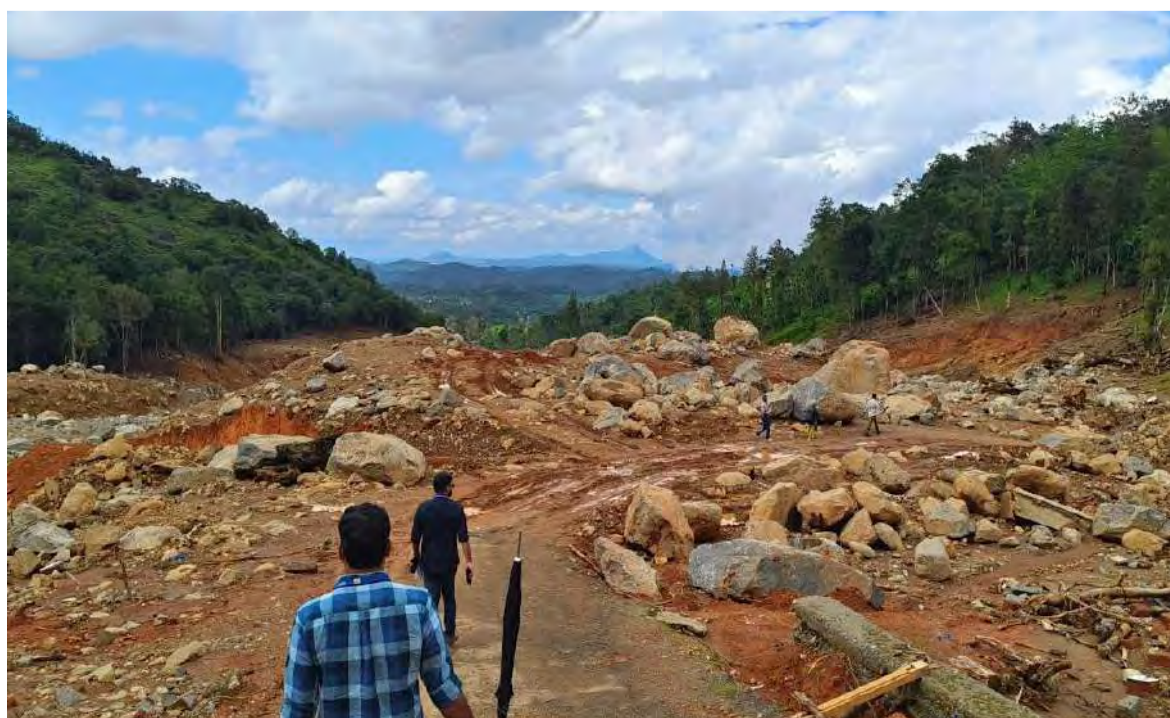
Figure 11-1: Meppadi landslide site
