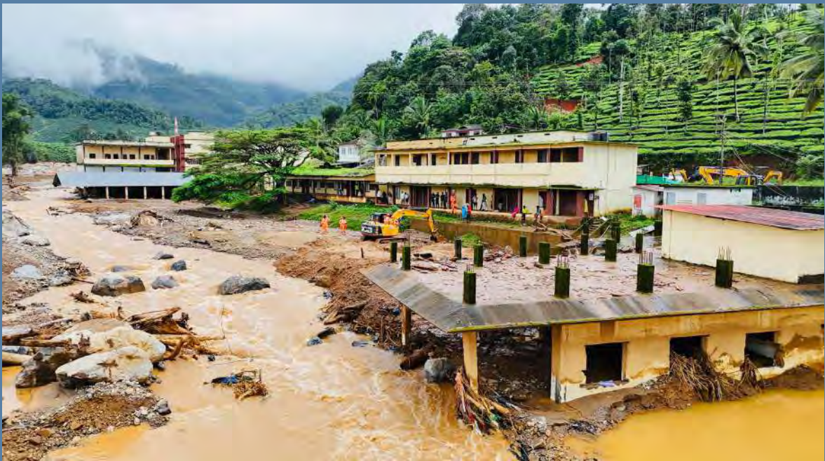
Figure 4-4: GVHSS Vellarmala after the Landslide
