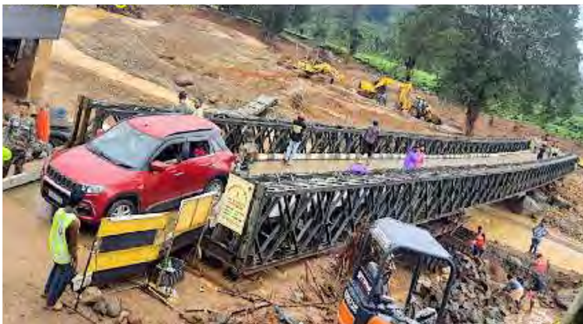
Figure 9-3: Bailey bridge constructed at Chooralmala by Army
