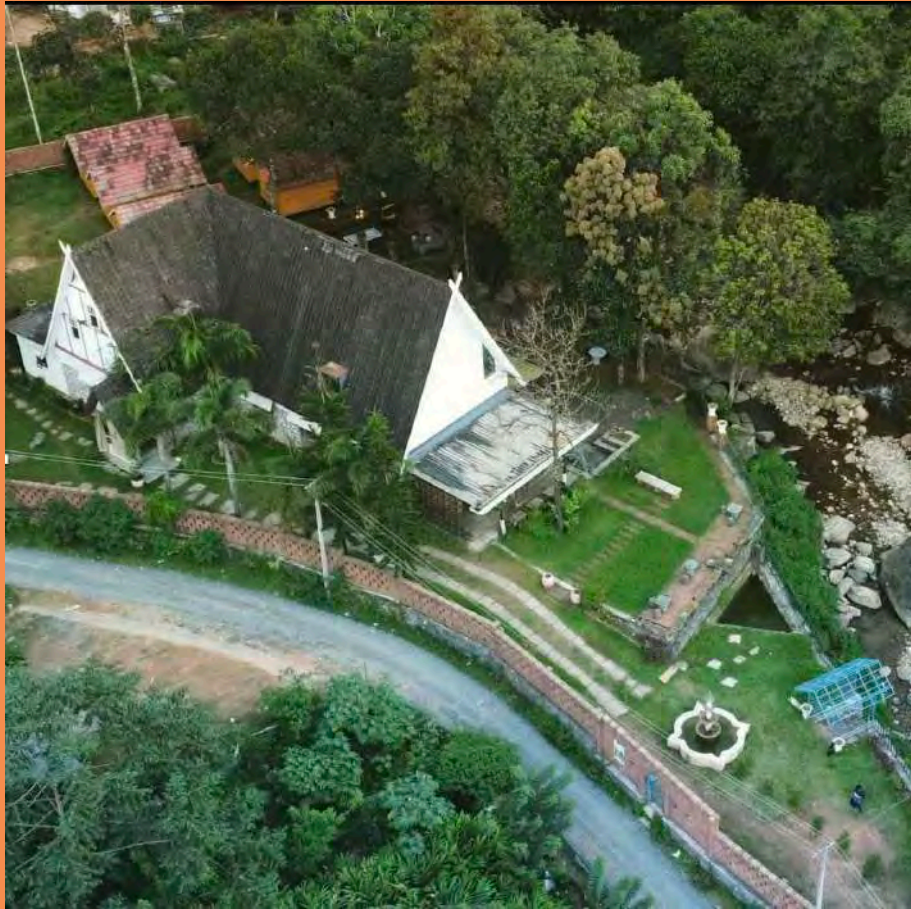
Figure 13-1: Preserve Stone Resort before landslide
