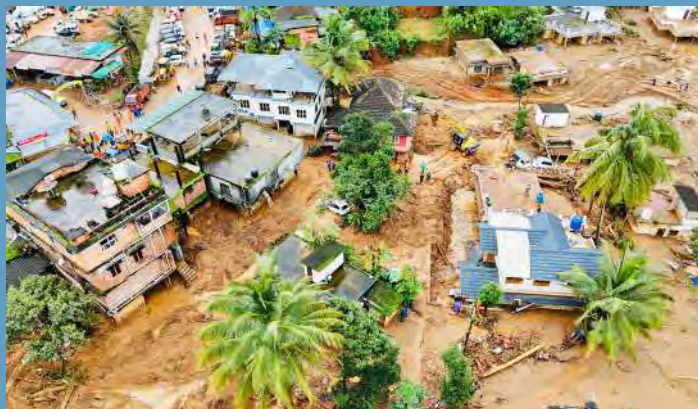
Figure 2-6: Houses affected by Meppadi landslide
