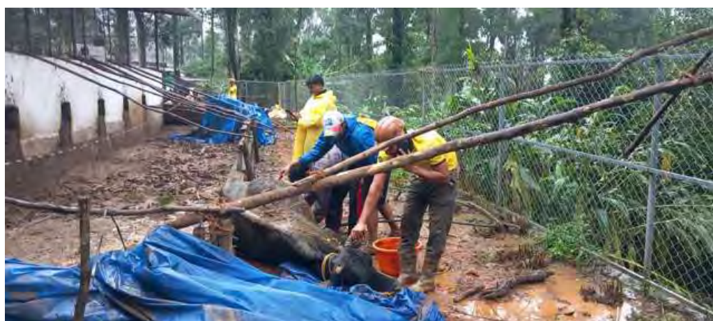
Figure 2-9: Damaged cattle sheds
