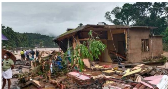
Figure 2-6: Photograph showing a destroyed house at Kootickal
