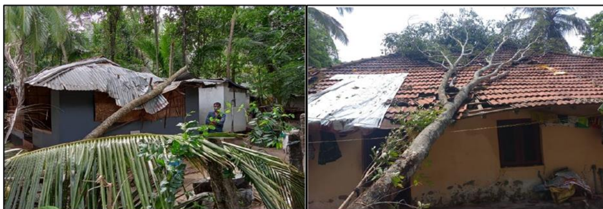
Figure 2-13: House damaged in Malappuram district due to Cyclone Tauktae (Source: District Emergency Operations Centre, Malappuram) (left); House damaged in Palakkad district due to Cyclone Tauktae (Source: District Emergency Operations Centre, Palakkad) (right) (Source: KSDMA)
