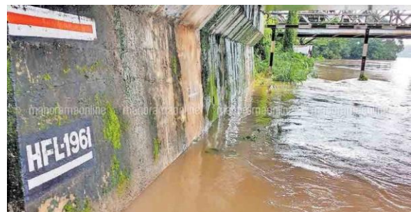
Water level marked at Chaliyar river below Feroke bridge during the 1961 floods
