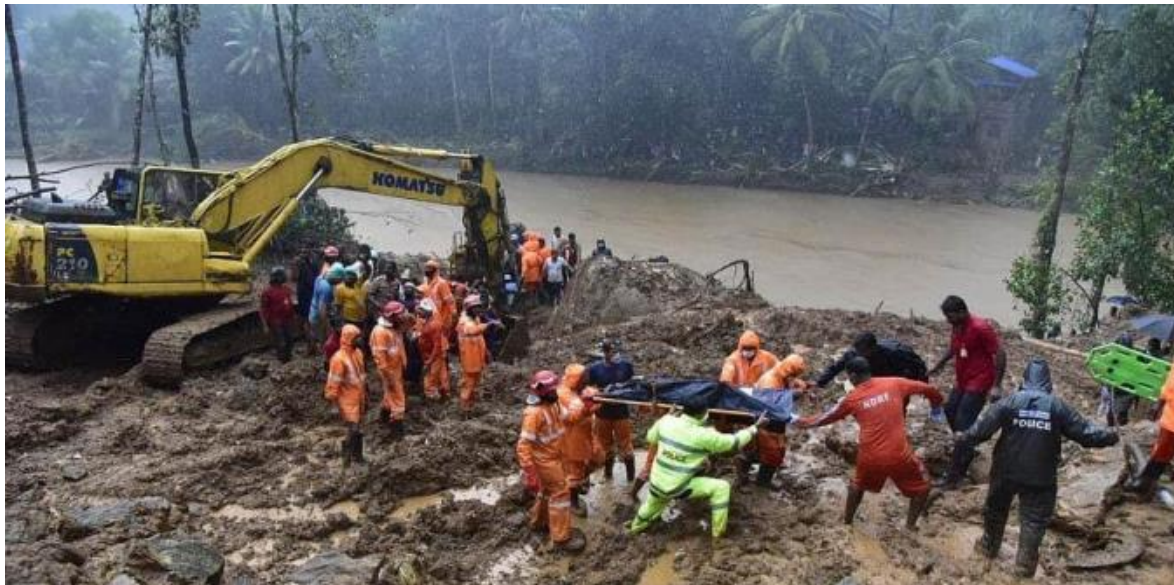
Figure 9-8: Rescue operations carried out at the landslide location near Mackochi in Kokkayar village
