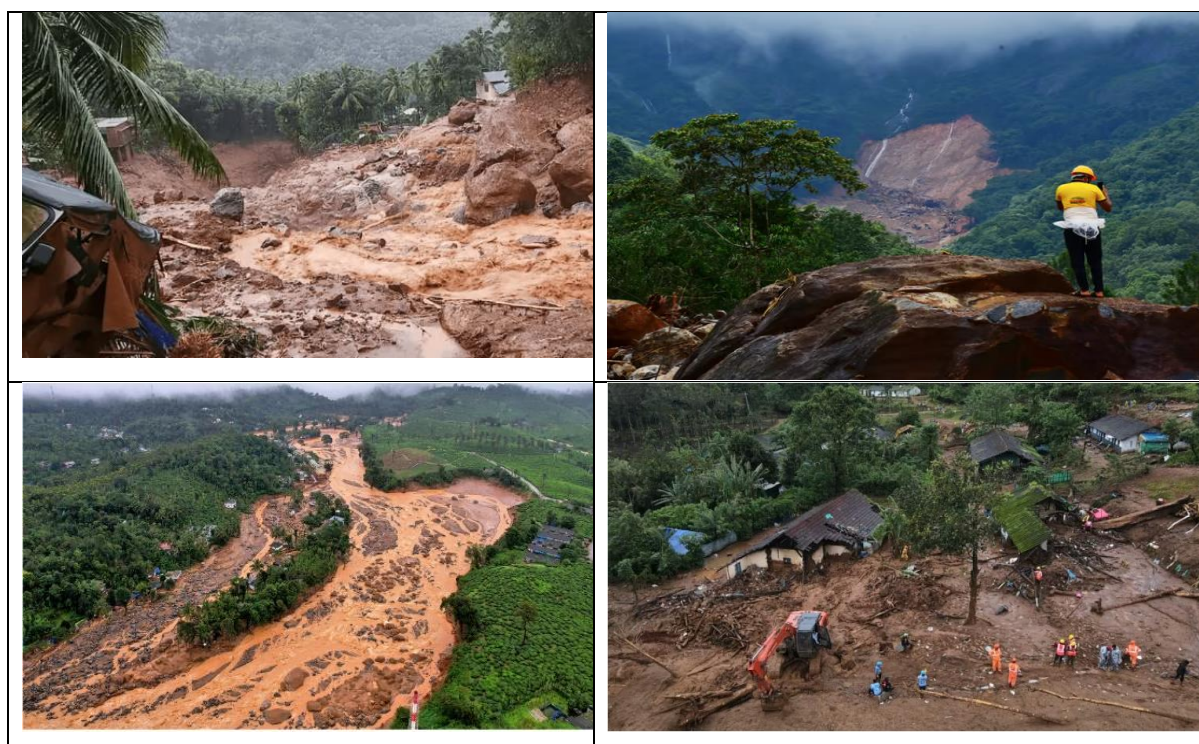
Figure 2-6: Some of the images from Wayanad post landslide event on July30, 2024
