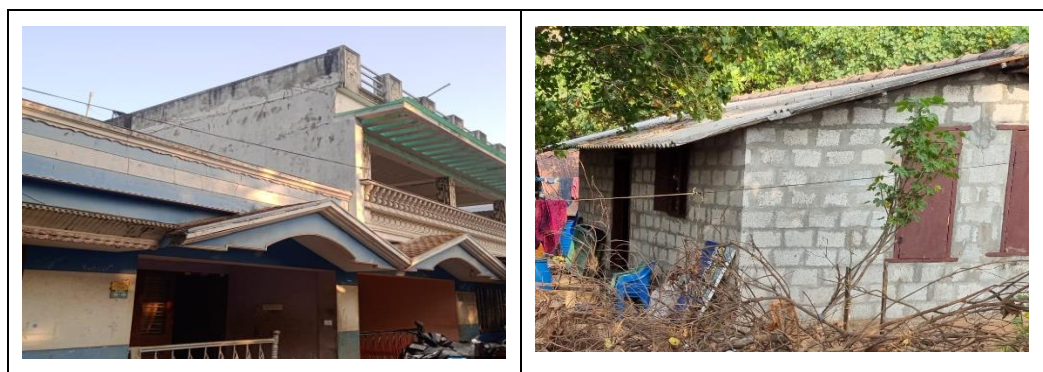
Figure 4-6: A few photographs of different type of buildings
