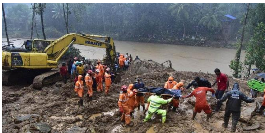
Figure 2-13: Rescue operations carried out at the landslide location near Mackochi in Kakkayar village
