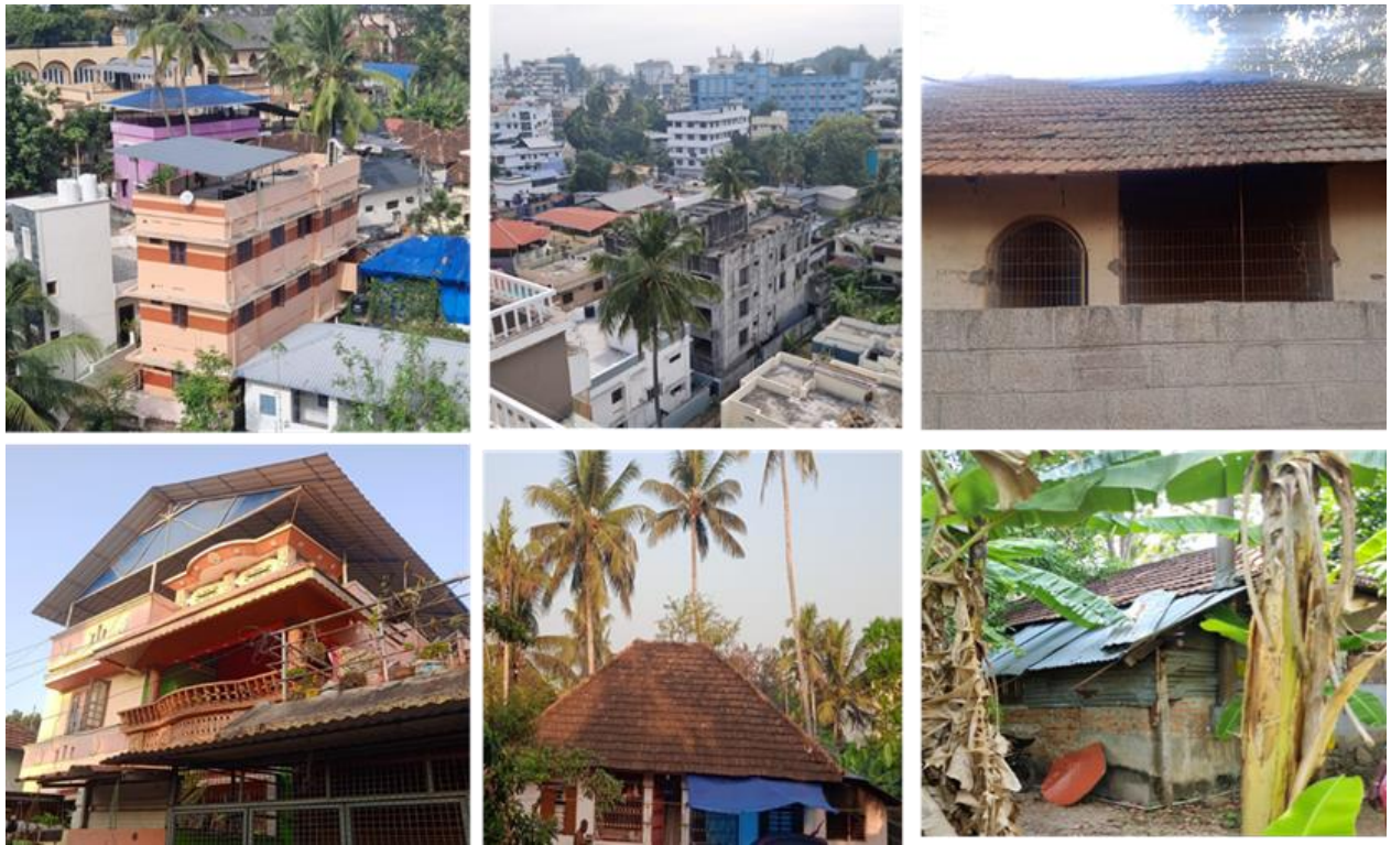
Figure 4-3: Building type photographs from field survey
